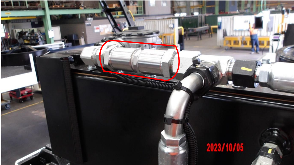
Figure 4 - Installing Replacement Assembly
