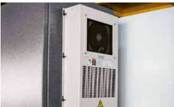
Heat Exchanger For Electrical Cabinet
